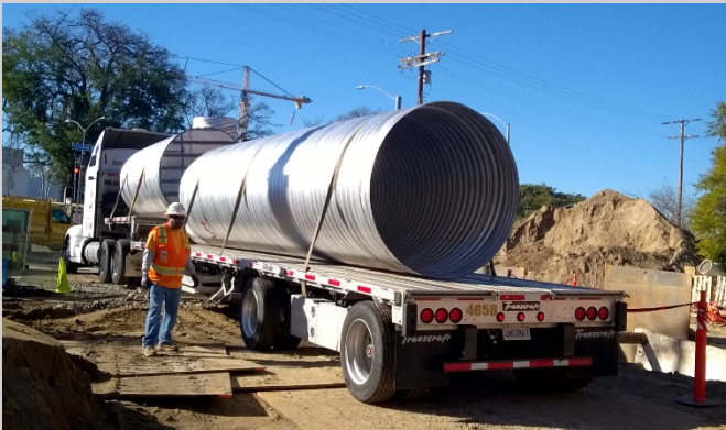
Stormwater detention piping being delivered to Watt Way
