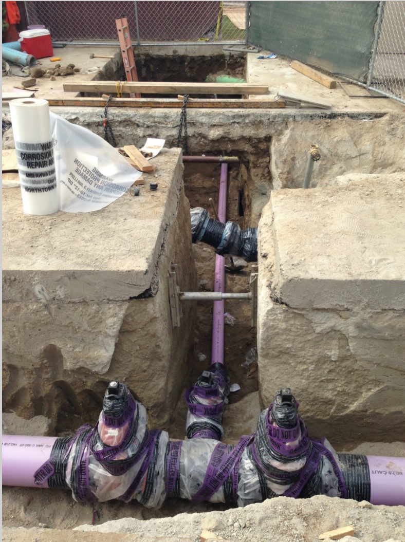
Recycled water piping install at McClintock Ave
