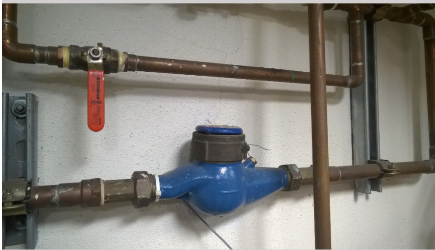
Interior water sub-meter
