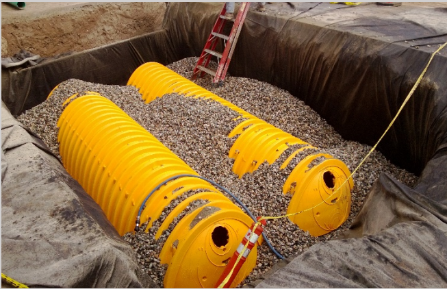
Underground Infiltration system at Robert Zemeckis Center
